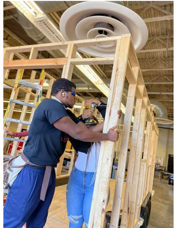
North Point student framing work Photo supplied by THinc
