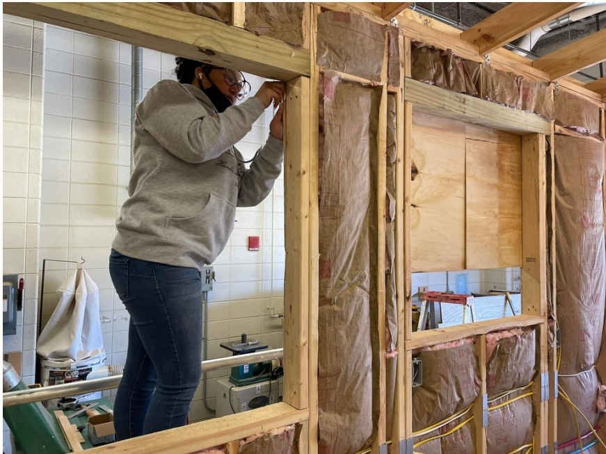
Construction in progress
